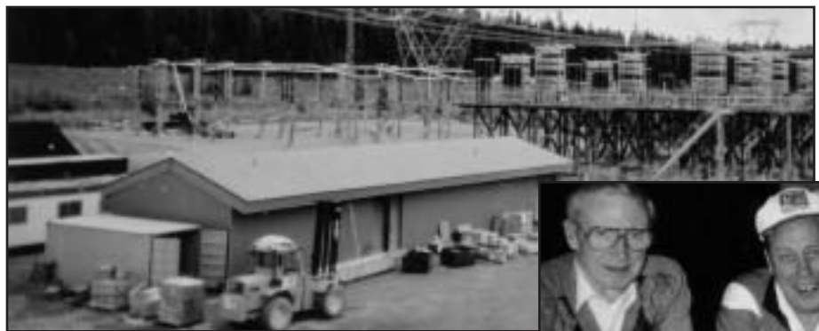
BC Hydro's McLeese Lake Capacitor Station Upgrade, near Williams Lake, June 2003.
